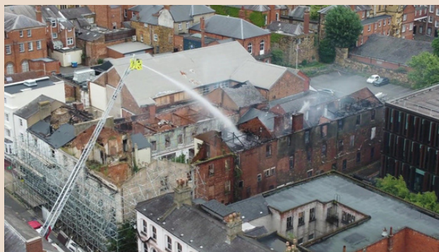
The Angle Hotel on Bridge Street burnt down in August 2023 and was demolished in September 2024.
